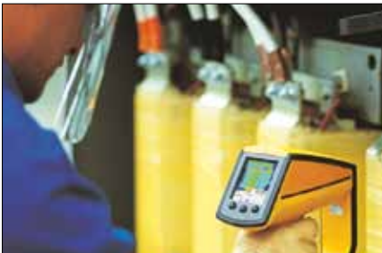
Transformer inspection
